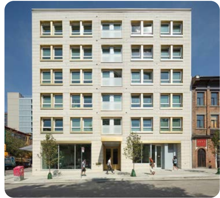
Example of a high performance building with human scale design that contributes to a high quality public realm, supports pedestrian activity and liveability for residents.
