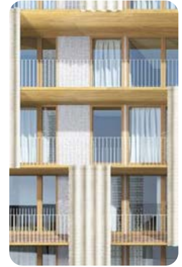
Examples of balconies located and designed to provide shade in summer and sunlight access in winter.
