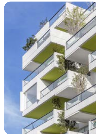
Examples of balconies located and designed to provide shade in summer and sunlight access in winter.
