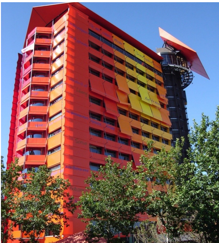
Strategy 1: Use external solar or security screens, shades or grilles, like these motorized solar shades.
